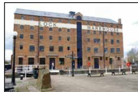
The newly restored Lock Warehouse.
