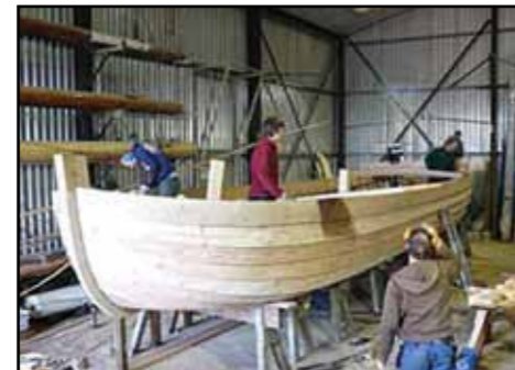
♦ The Trow under construction in Tommi Nielsen's shed.
